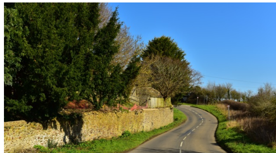
Expectations for strategic network road condition are for a higher standard with no running lane defects and a smoother ride quality.
